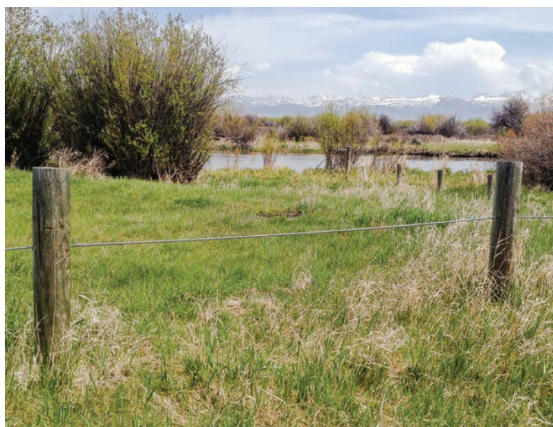
A post fence with a single cable or chain between posts can also mark a boundary yet give wildlife free passage. Credit: Christine Paige.
