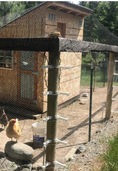
Chicken coops and beehives are irresistible to bears, but high-energy electric fence is effective protection. Credit: Tim Manley.
