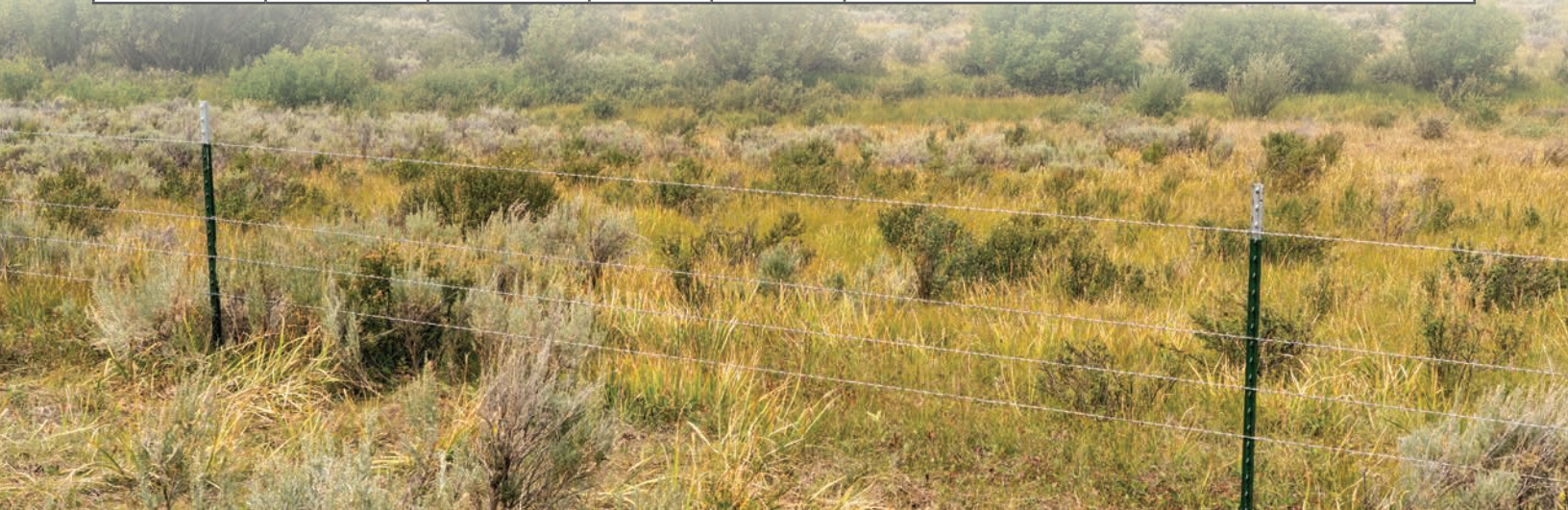
A friendlier wire fence with smooth bottom wire and 12" gap between top and second wires. Credit: Christine Paige.
