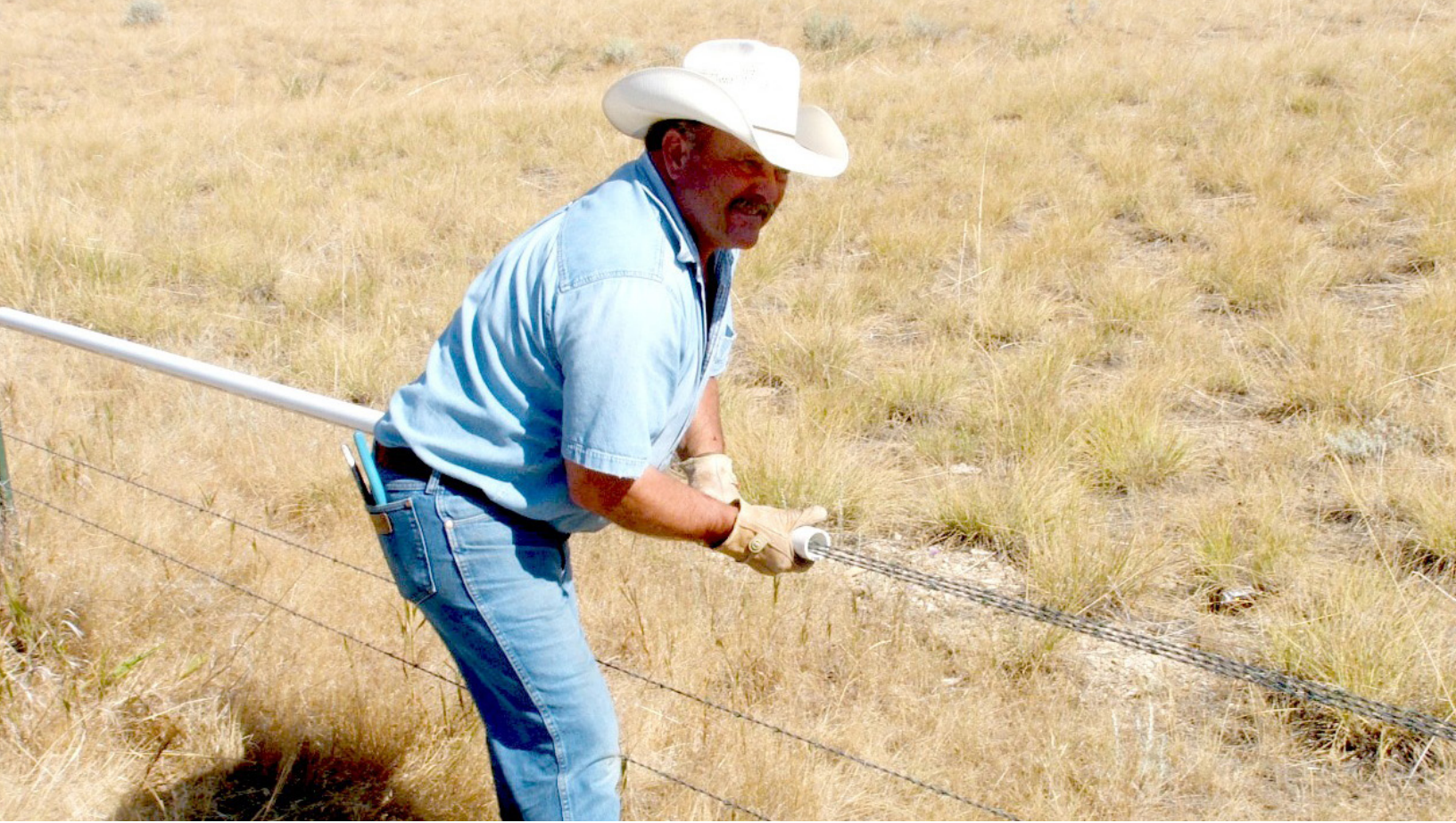
PVC pipe threaded over bunched fence wires and quick links to gather bottom wires can create a durable big game passage, especially on road rights-of-way. Credit: Montana Fish, Wildlife and Parks.
