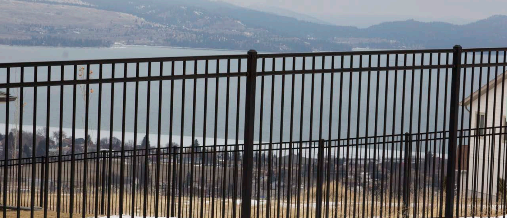
A solid top rail and narrow vertical bars on this iron fence reduce hazards to wildlife. Bars should be spaced less than 6" apart so fawns aren't trapped if they try to press through. Credit: Christine Paige.
