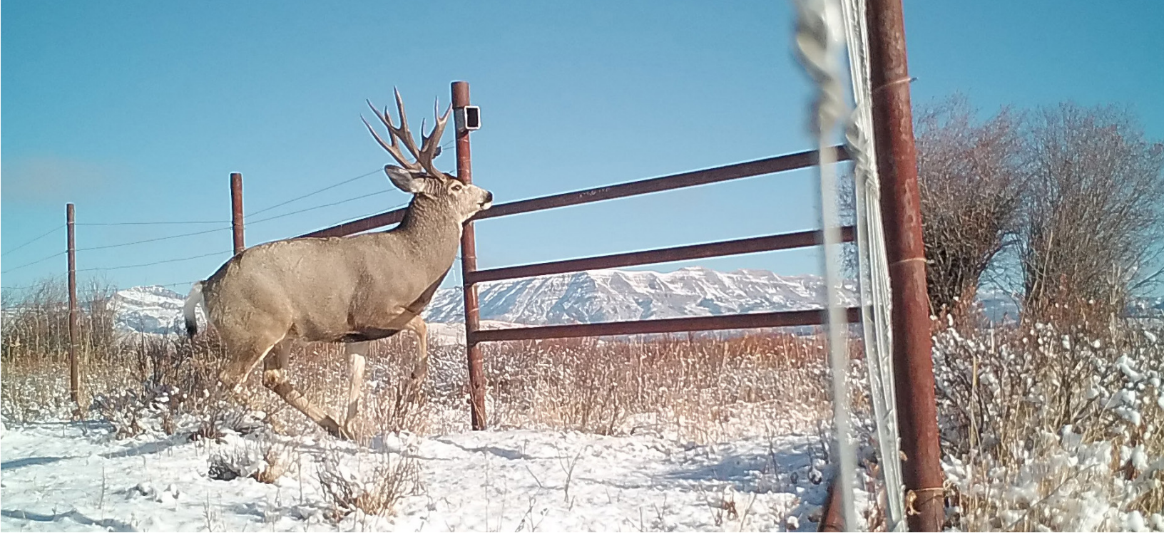
Wyoming Game and Fish Department tested wildlife jumps in bison fence near Bondurant. The jumps were built with welded pipes at 16-18," 30," and 40" with a removable top rail at 60." During spring and fall migrations, the top rail is removed, making passage easier for elk, deer, and moose while still containing bison and excluding nearby cattle. Credit: WGFD.
