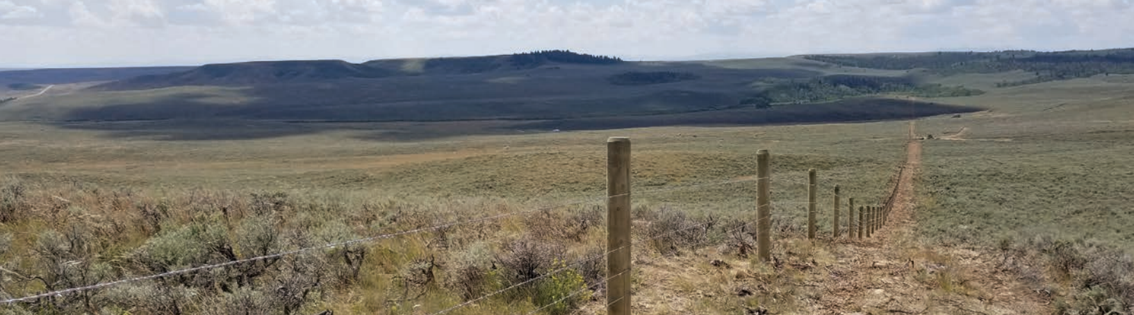
This 4-wire wildlife-friendlier fence was installed within the Sublette Mule Deer Migration Corridor as part of the Upper Green Fence Initiative. Credit: Troy Fieseler, WGFD.
